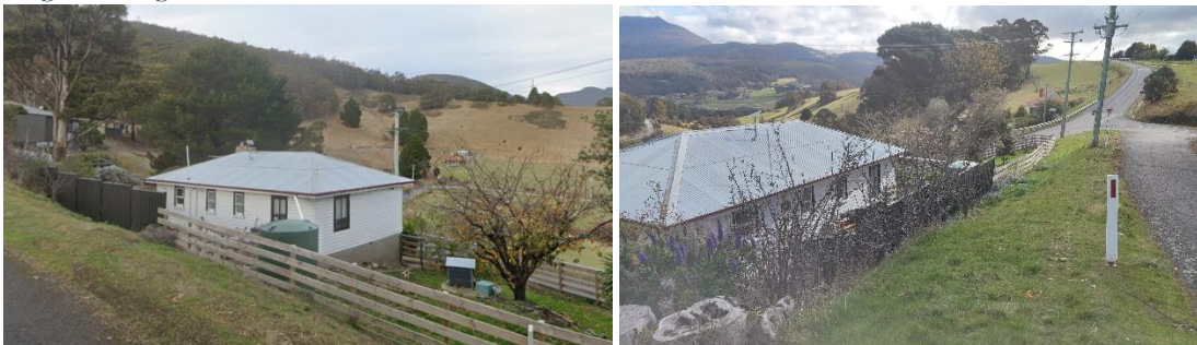
Figure 1 View of existing residence from Collinsvale Road
