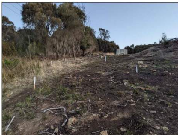
Figure 9-5 Prop. access, Ch300-335m
