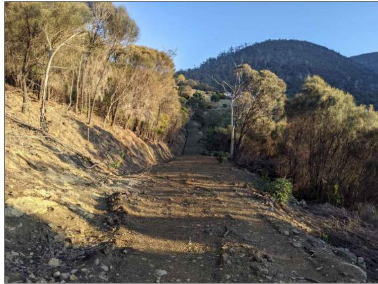
CH170 LOOKING TOWARD CH000 PULLOVER BAY LOCATION
