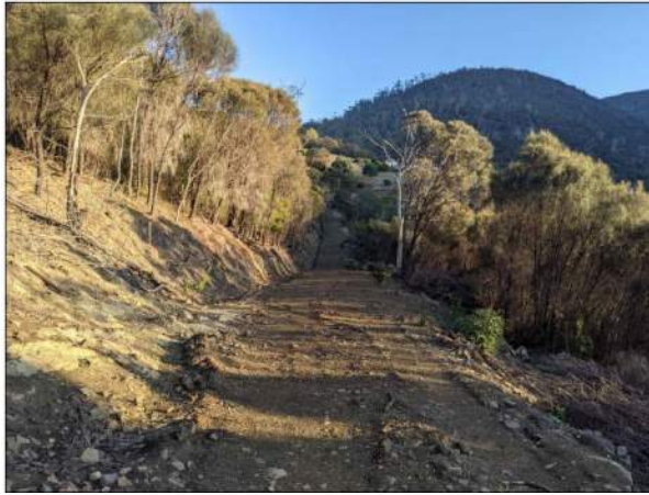
Figure 9-1 Existing access, Ch170m
