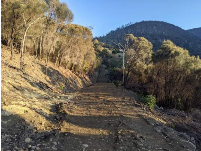
Figure 2: FORMED DRIVEWAY: CH000 – CH190
