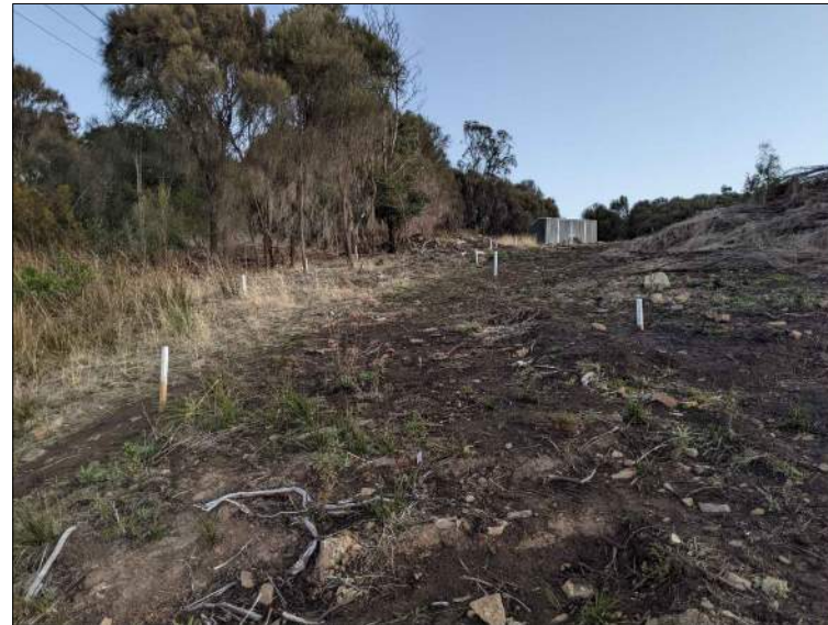
CH300 TO CH335 CLEARED SECTION
