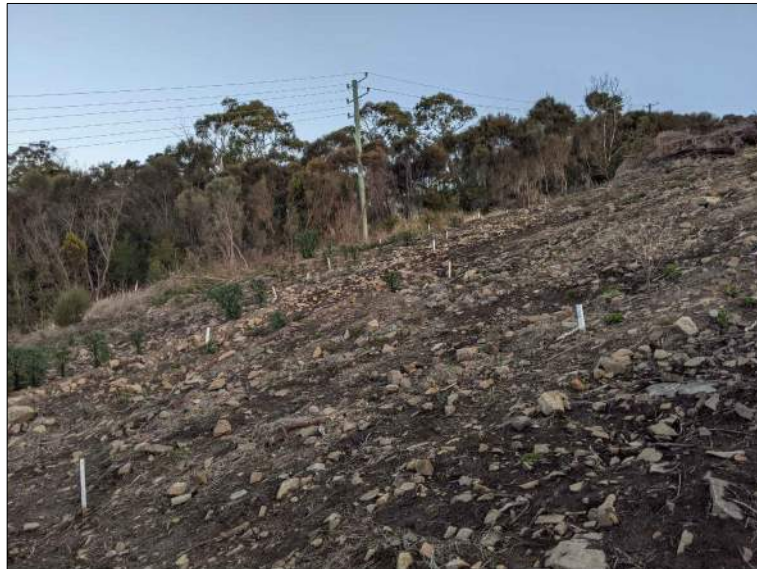
CH270 TO CH300 CLEARED SECTION
