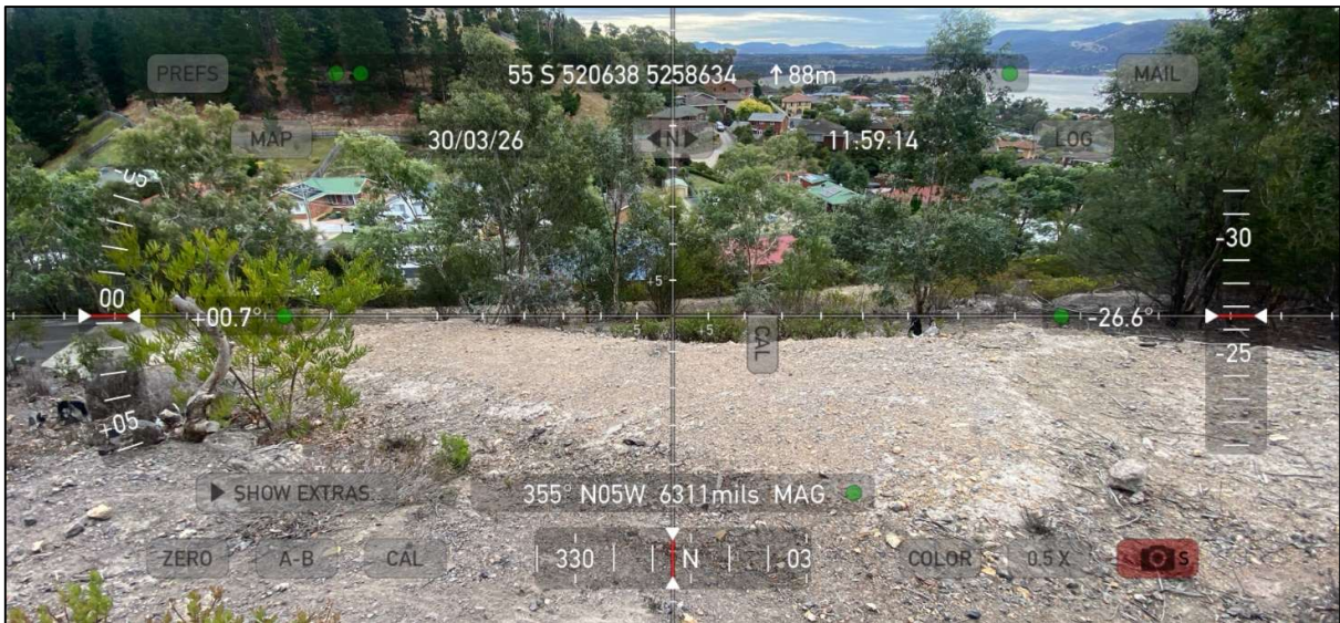
Image 9 – Proposed building area viewed from the south
