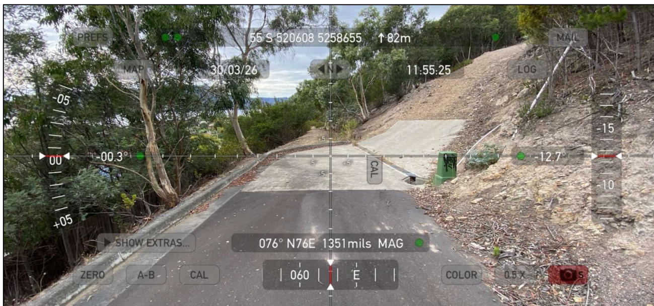
Image 6 – Termination of existing independent access to the subject land, forming the basis for a compliant ‘Y’ turning area and hardstand, with a static water supply for firefighting to be located at the upper left of the image
