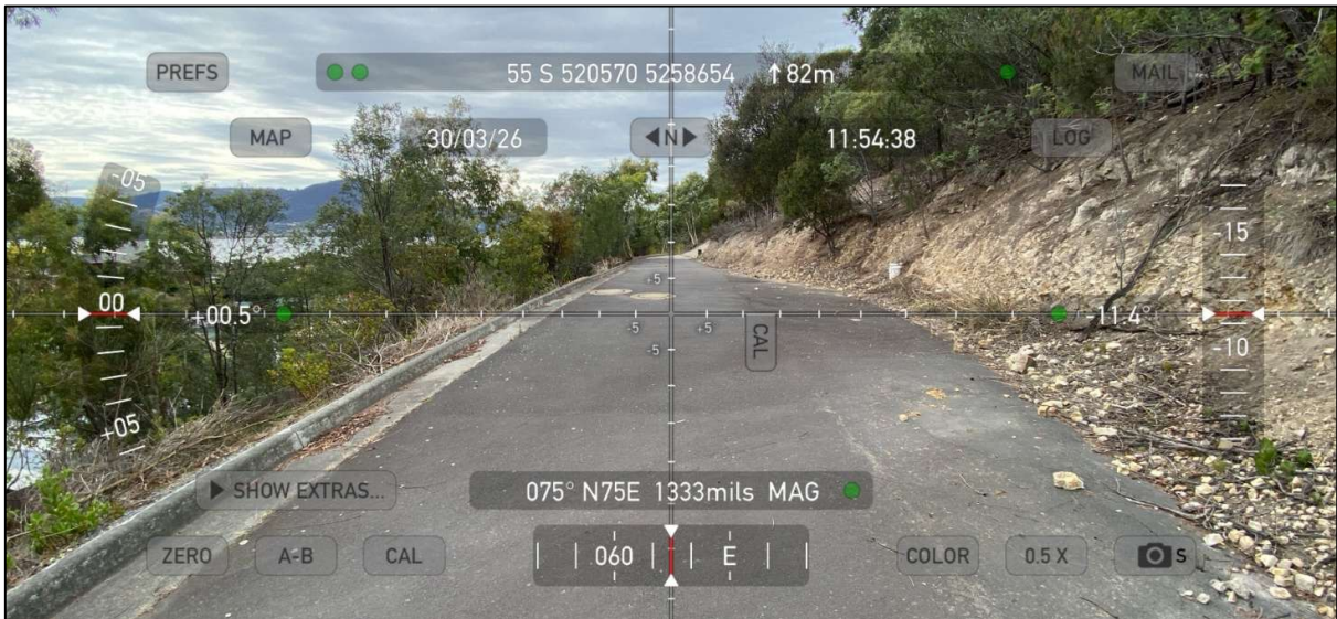
Image 5 – Upper section of existing independent access to the subject land
