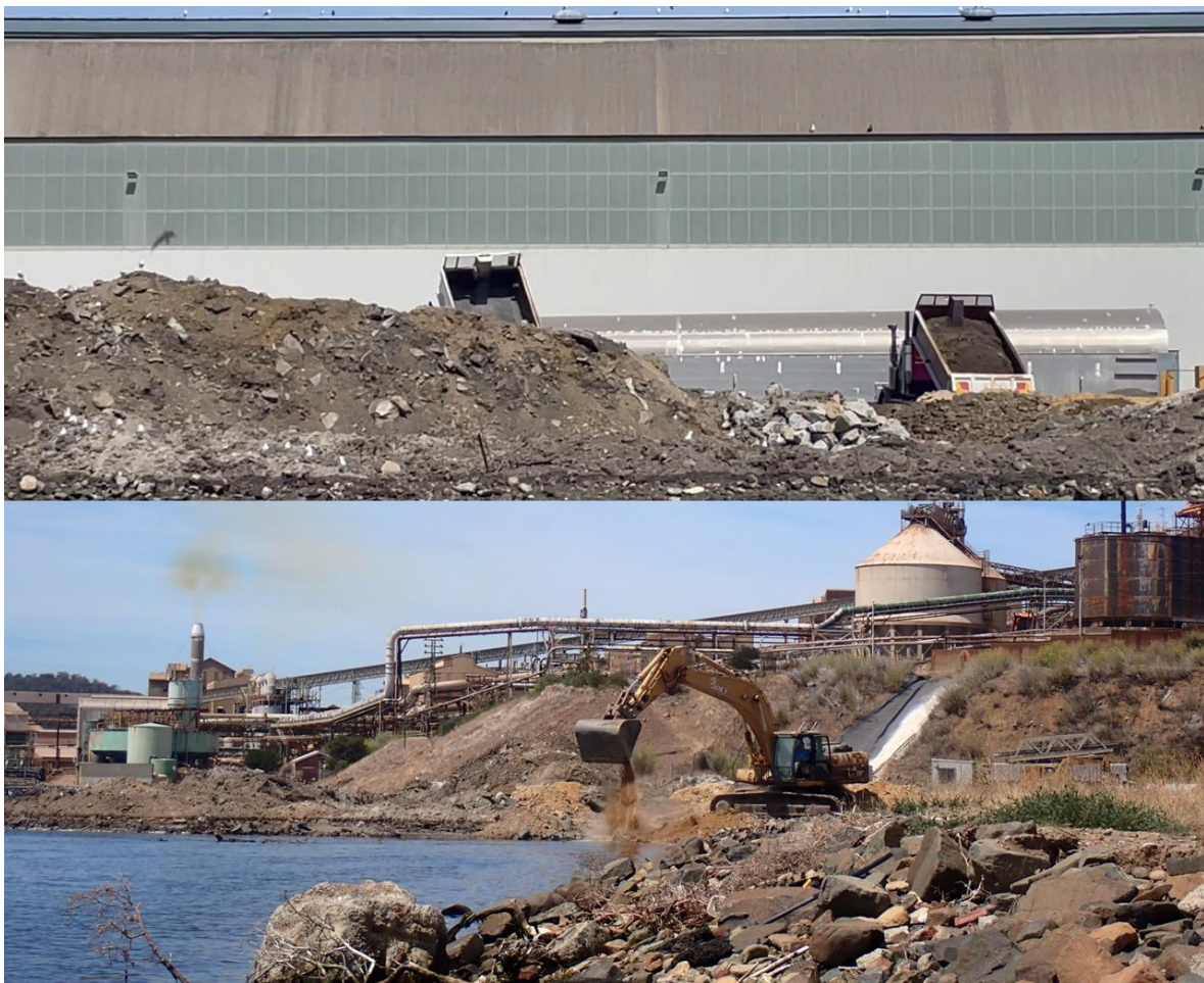
Figure 4 Reclamation works in progress on 3 February 2026, including fill delivery by trucks (top) and sediment placement into the River Derwent (bottom).
