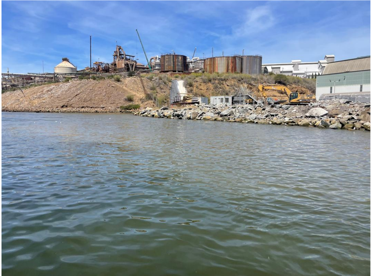
Figure 5 Significant sediment plume surrounding the construction and reclamation site, taken from survey vessel by field personnel on 3 February 2026.
