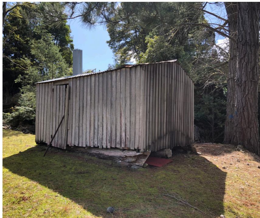
SMALL HUT - EXISTING EXTERNAL PHOTOS
